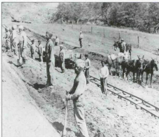
Sikh workers from the Punjab region of India construct a section of the Oregon Pacific & Eastern Railroad, which serviced the lumber industry, c. 1909. (Courtesy of the Southern Oregon Historical Society, #1603)
